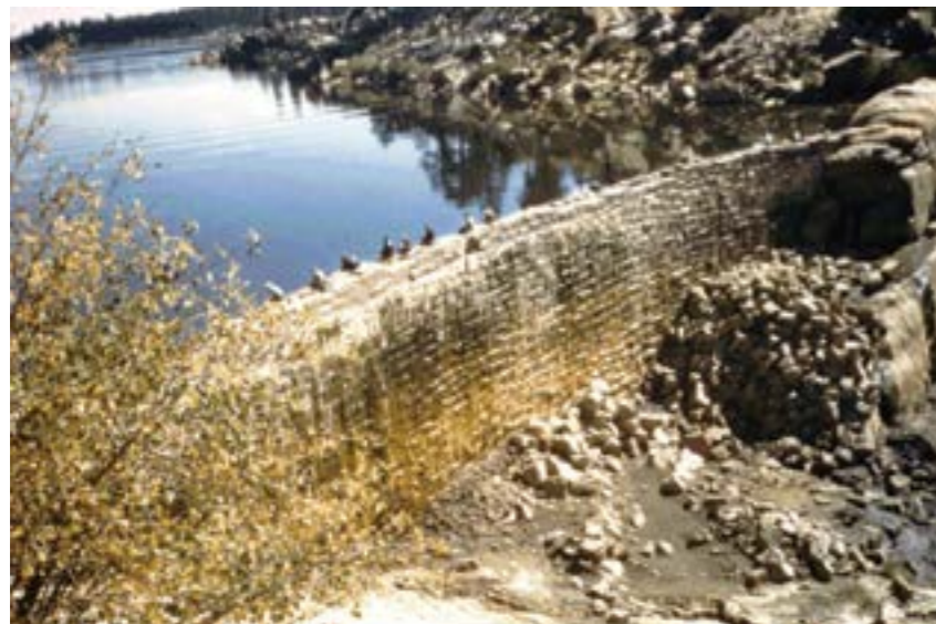
Completed in 1884, the original Bear Valley Dam was the world's first arch dam
